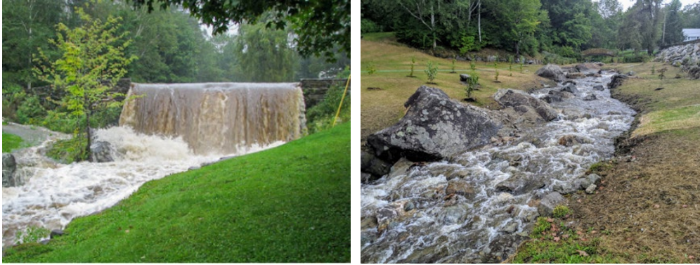
Figure 35. Before (left) and after (right) the removal of the Cold Spring Brook Park dam in the Town of Weston, which restored over 351 linear feet of stream and reconnected 0.2 acres of floodplain. Project funded by a DEC Clean Water Initiative Program grant. (Source: Weston Community Association)
