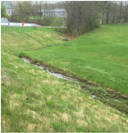
Figure 30. Before (left) and after (right) the conversion of a paved swale into a gravel wetland to treat runoff from the parking lot at the Hazen Union School in Town of Hardwick. Project funded by a DEC Clean Water Initiative Program grant. (Source: Caledonia County Natural Resources Conservation District)
