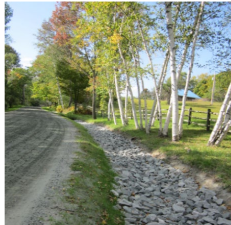
Figure 31. During (left) and after (right) the construction of stone-lined drainage ditch in the Town of West Windsor. Project funding provided by VTrans Better Roads Program. (Source: VTrans)
