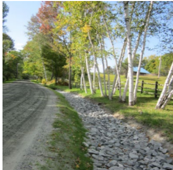
West Windsor drainage ditch improvement funded by Agency of Transportation Better Roads Program
